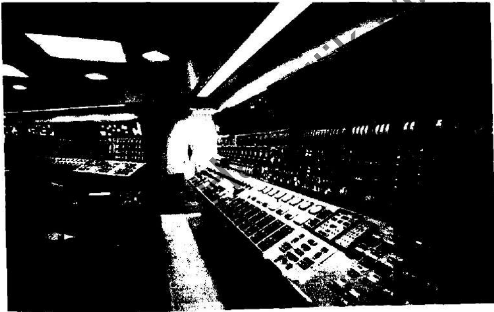
Figure 10: Tunku Jaafar Power Station Port Dickson
