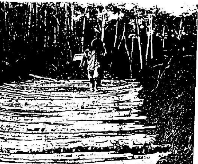
Fig.5. Tree trunks used to stabilize the base of a road on soft soil in the tropical jungle.
