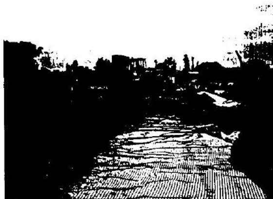
Fig.32: TENAX GT geocomposite provides separation between the base and the subgrade, and tensile strength and lateral confinement to the fill.
