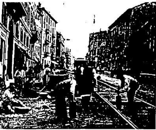
Fig.3: Installation of cobble stones and kerbs in the main road Corso Venezia, Milan (Italy), 1920 ca.
