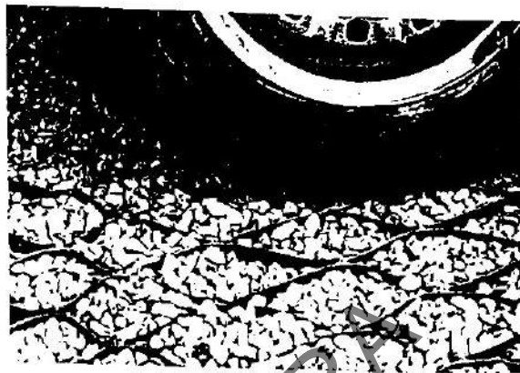
Fig.31: TENAX TENWEB geocells provide the lateral confinement required to reduce the thickness of aggregate to a minimum.
